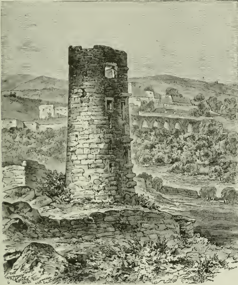
GREEK TOWER AT ANDROS. 1
